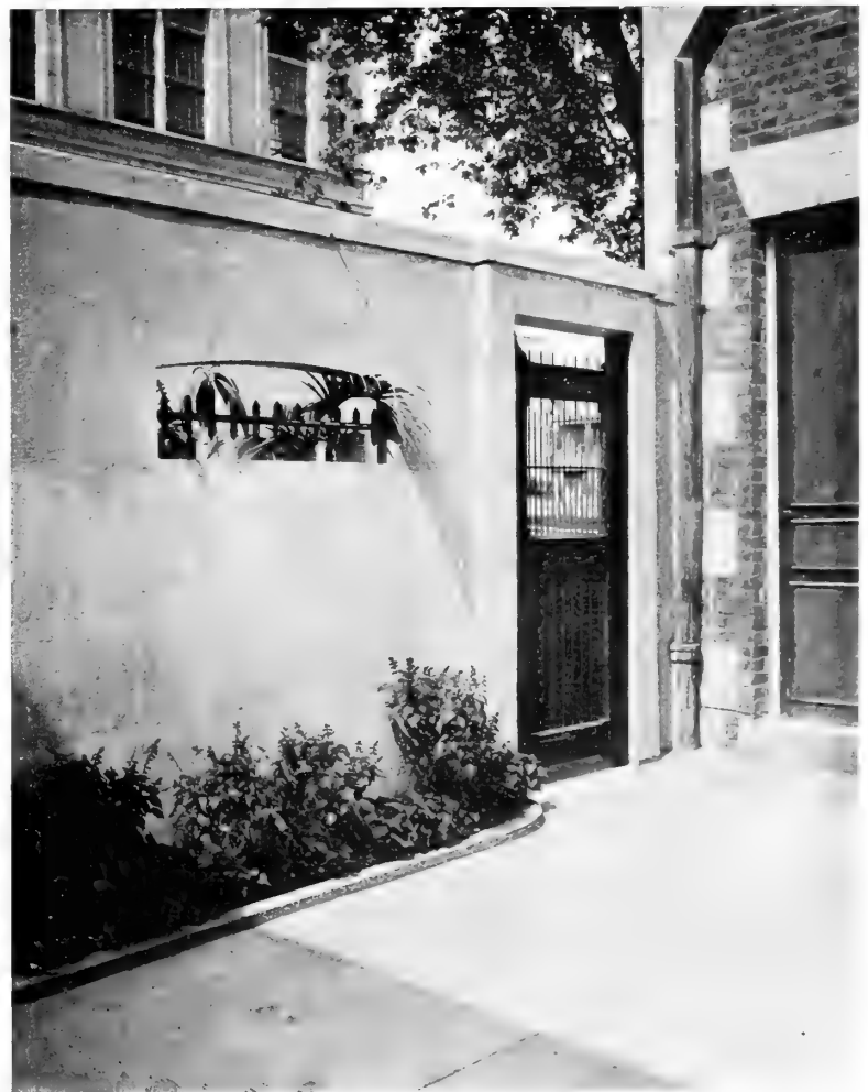
The Gateway from the Street to the Court, and the Wall Built of Reinforced Concrete
